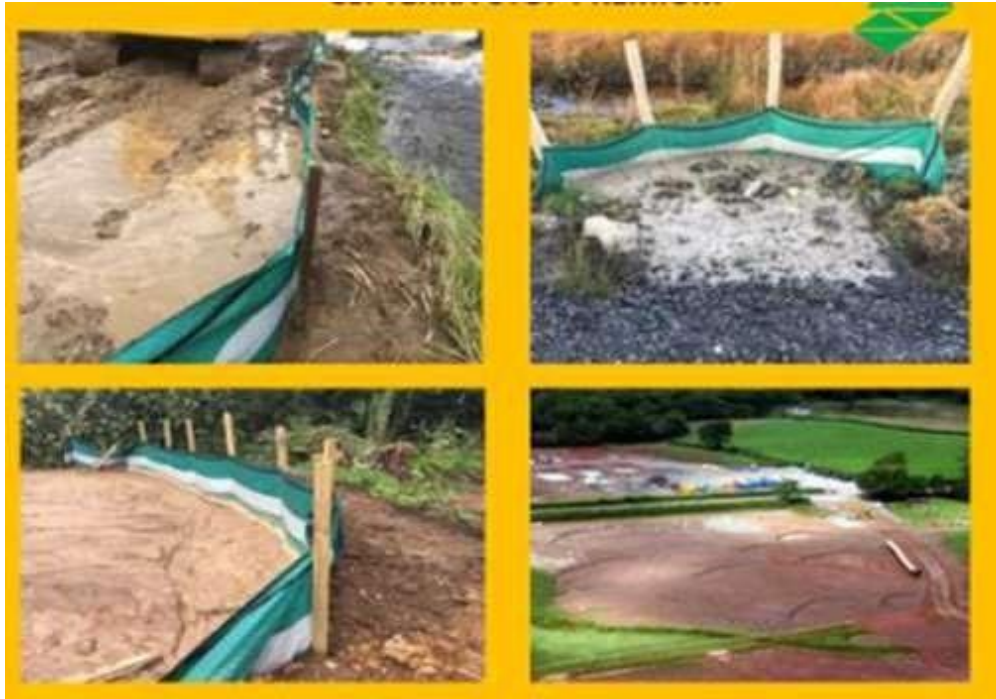
Plate 9 Silt fencing.
